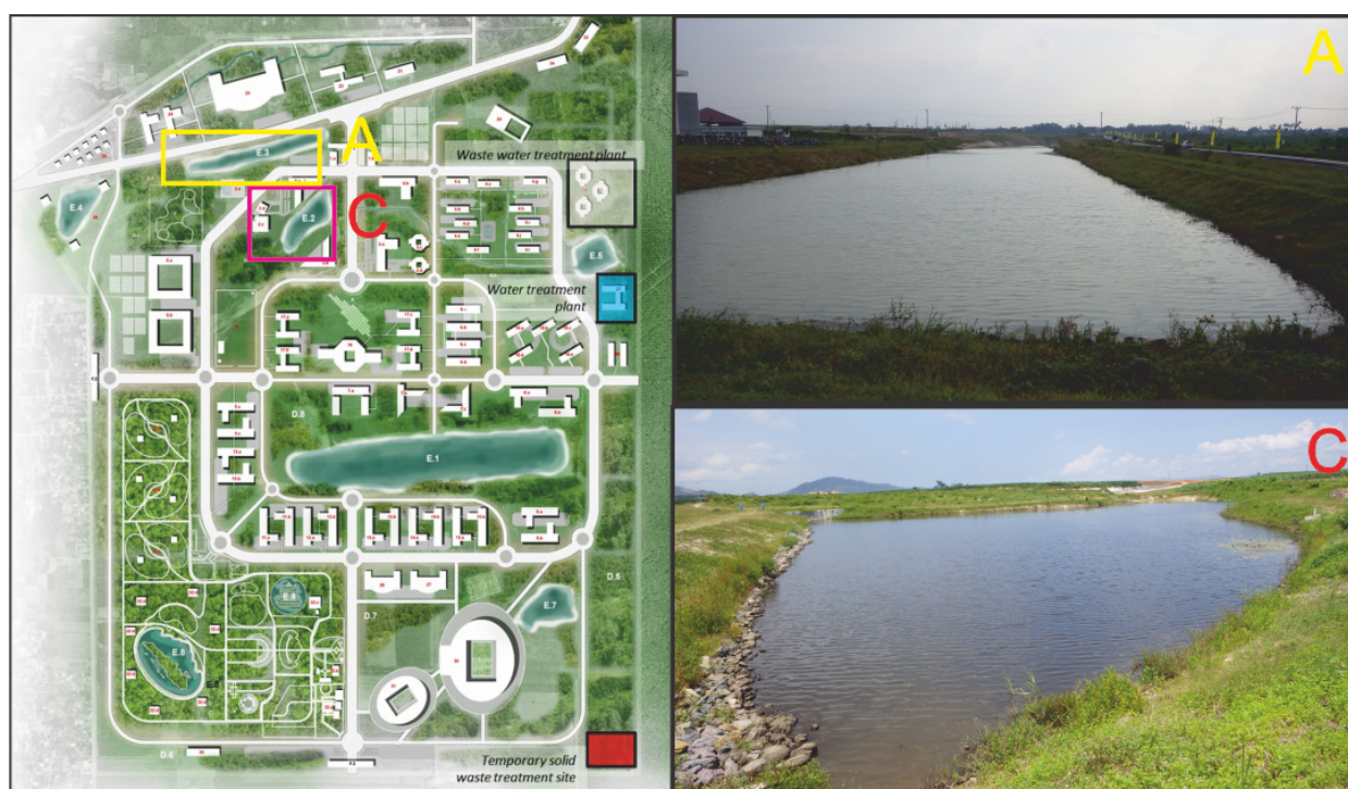
Figure 1. Location of Pond A and C of ITERA in 2017. The pictures were taken in May before construction.
