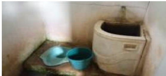
Figure 1. Condition of Sanitation
