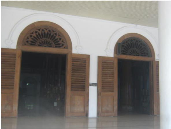
Figure 2. Large size doors and vents for good air circulation
