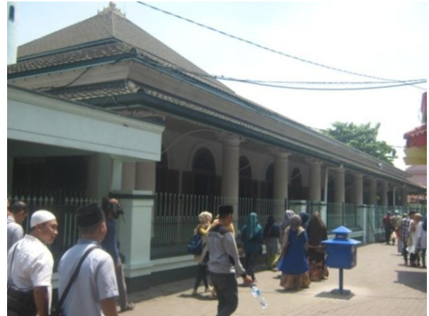
Figure 3. The original part of the building with circulation for visitors
