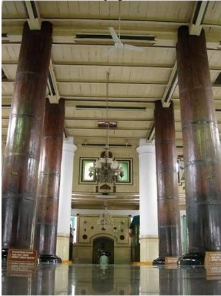
Figure 7 The main hall of the Great Mosque of Demak with four main pillars ( soko )
