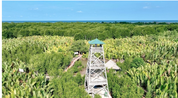
Figure 2 Mangrove Monitoring Tower Facilities
