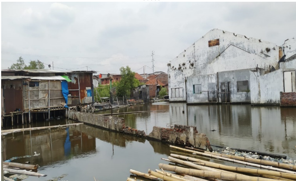
Figure 6. Land subsidence made residents of the Bandarharjo sub-district required to fill in and elevate their houses
