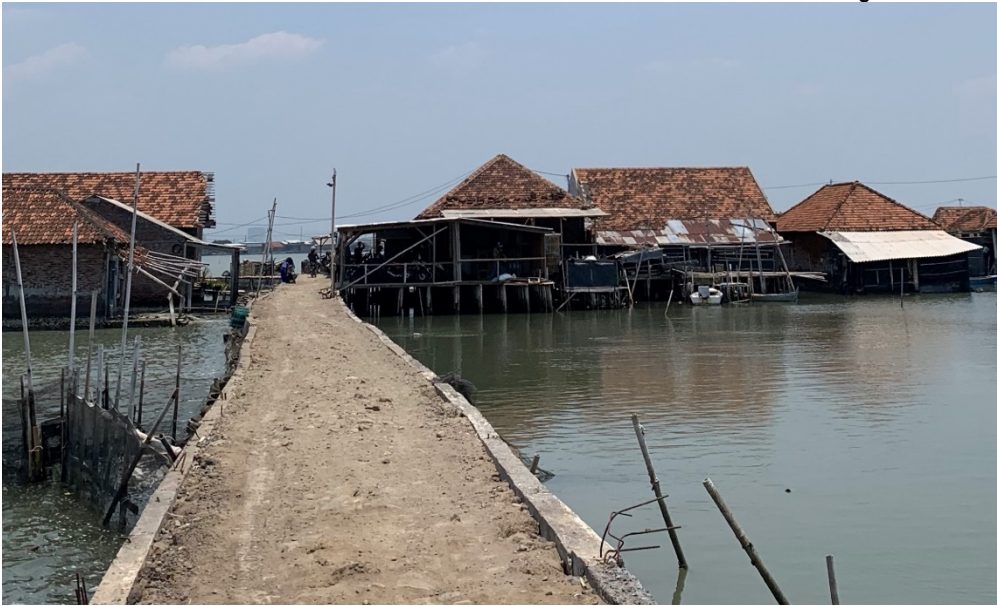
Picture 2. Main road access to Timbulsloko Hamlet, Timbulsloko Village
